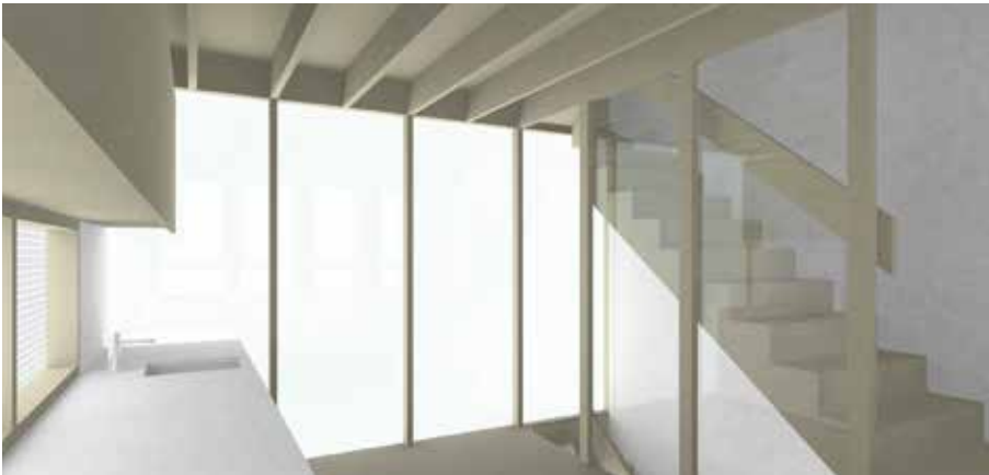
Thermally broken frames with high-performance double glazing has lower embodied carbon than a triple-glazed system over the life of the building.
